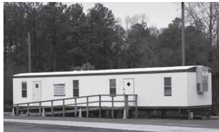
It aint pretty but its home for now. This is the temporary visitor contact station that will serve visitors while the National Prisoner of War Museum is closed for maintenance.
